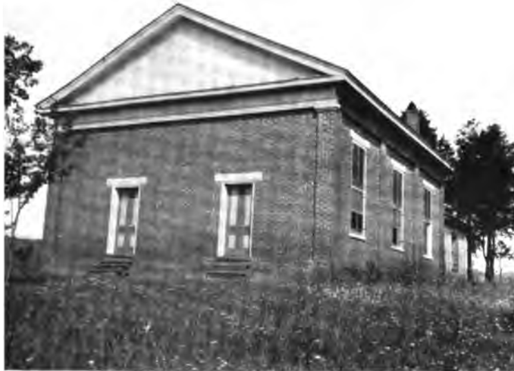
(A) Church constructed of brick made from local clay and erected before the Civil War.
